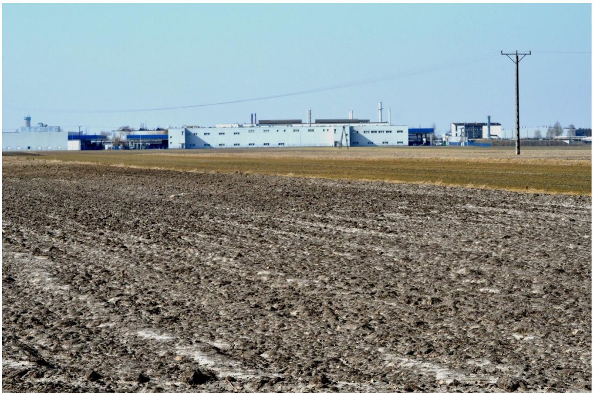
a view from Spartańska street (a view from the South)
